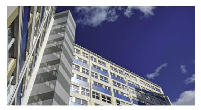
Wilmcote House is an 11-storey residential development in Portsmouth. Built in 1968, its original structure comprised of large, poorly insulated concrete panels with precast concrete elements that significantly bridged the thermal envelope, leading to high heat losses, internal condensation risk, mould growth and low internal comfort standards.
