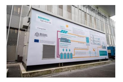
Siemens installed electrical energy storage at MMU Business School to enhance the energy efficiency as part of the Triangulum project, enabling excess electricity to be stored and used at times of peak demand.
