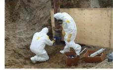
Canadian Nuclear Laboratories carrying out a pipe sealing operation on an active pipe using a bespoke FOAMBAG™ kit designed specifically for their project
