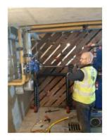
A new connection being made under live conditions using our under pressure system
